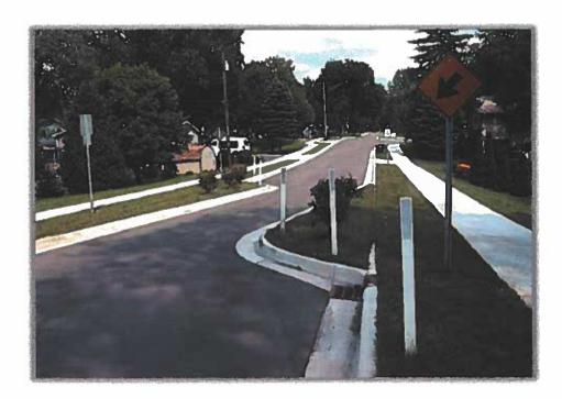
Neck-Downs – Physical modifications to the roadway that reduce or eliminate excessive pavement areas in order encourage slower speeds. Neck-downs can be constructed from either the center of the roadway or from the outside (shoulder side) of the roadway, or both. Neck-down are often used in combination with chicanes or neighborhood entry features.
