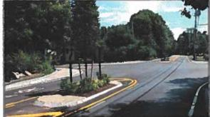
Chicanes – Physical modifications to the roadway that use a combination of horizontal curvature and lane narrowing to reduce speed, often creating a slalom effect. Chicanes can either maintain two-way traffic with narrowed lanes or can reduce pavement width to allow for only one-way traffic time.
